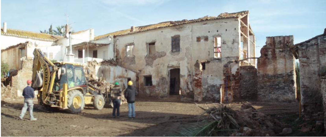
The building at the beginning of the intervention
